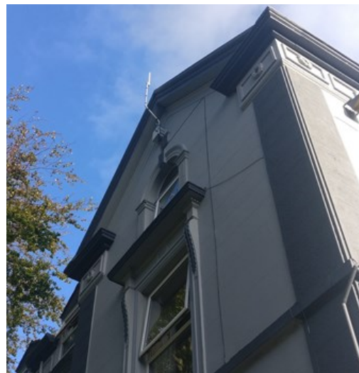
Completed gateway mounting at Breckside Park Care Home
